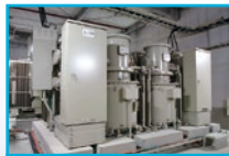
66/77kV Gas Insulated Switchgear (Indoor Type)
