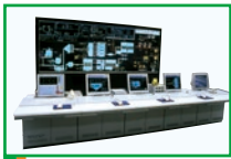
Supervisory Control System for Waterworks
