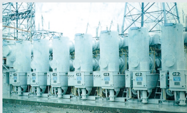
Three-phase integrated GIS
