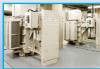
22/33kV Spot Network Substation Equipment
