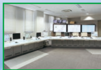
Supervisory Control System for Expressways
