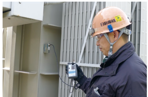
On line inspection using a partial discharge detector
