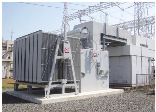
図3 ShR 33kV 60MVA 65dB(A)
