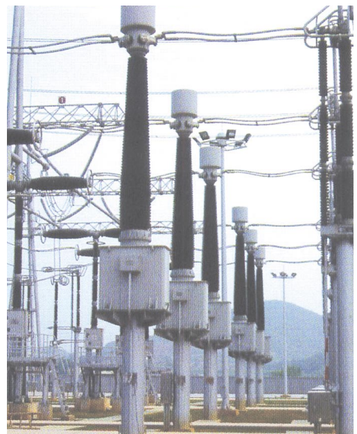
Fig. 11 500 kV Hair-Pin Type CT
