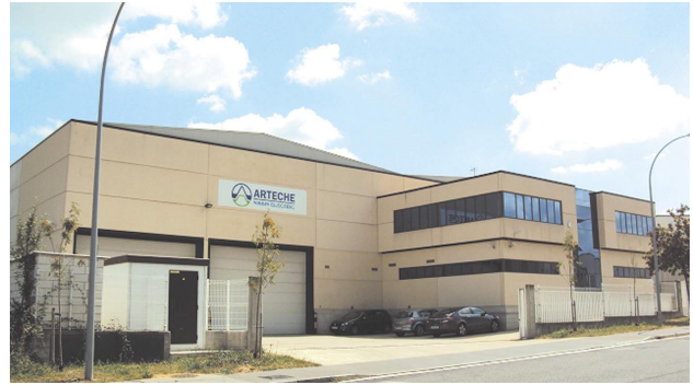
Fig. 30 ANSL's Plant in Spain
