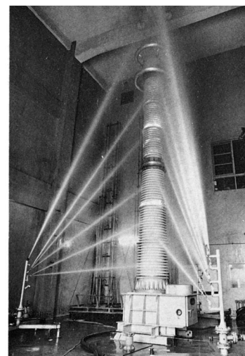
b) Washing withstand voltage test
