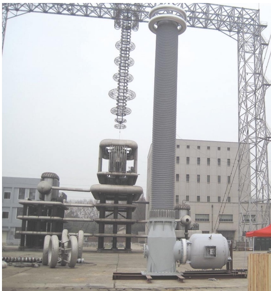
Fig. 19 Operation Test of 1,100 kV Gas VT
