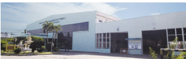
Exterior of the new factory at Nissin Electric (Thailand)
