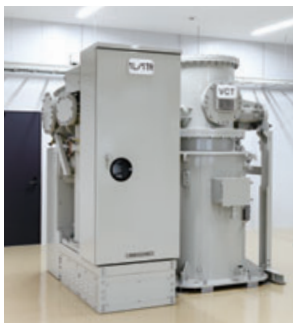
3 GIS Practical Training Room
