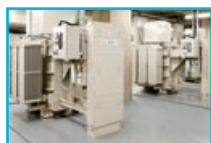
22/33kV Spot Network Substation Equipment
