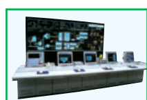
Supervisory Control System for Waterworks
