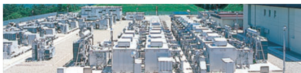
66/77kV Harmonic Filter Equipment
