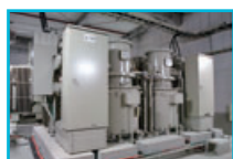
66/77kV Gas Insulated Switchgear (Indoor Type)
