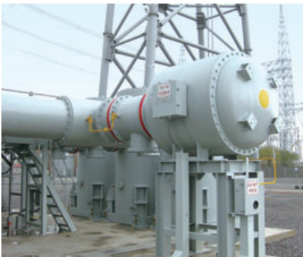
1,000kV Gas Insulated Voltage Transformer (UHV VT)
