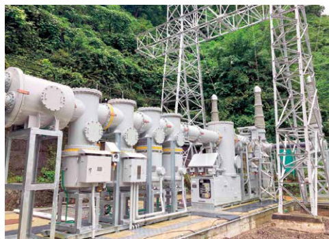
図1 168kV 縮小形GISとGIS直結形VCT
