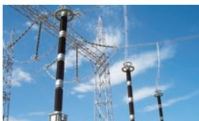
Capacitor Voltage Transformer (CVT)
