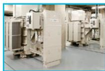
22/33kV Spot Network Substation Equipment
