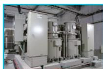
66/77kV Gas Insulated Switchgear (Indoor Type)
