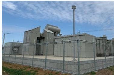
Passive filter for harmonic resonances measures for wind power generation
